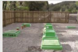
▶ Example of a fully installed 50PE Novo wastewater treatment unit in a 5-star hotel.
