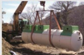
▶ Each WWTP unit is constructed of lightweight SMC and is easy to maneuver which simplifies the installation process.
